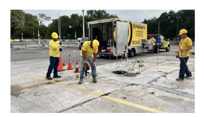
Inject chemical grout up to 10 feet in depth to solidify and stabilize the soil. The chemical grout was injected directly under the slab to compress the top layer of soil while stabilizing the slab. The quick cure time of the chemical grout allowed the area to be able to support loads almost immediately. All operations at the Waste Management facility were up and running and back to normal in no time.
